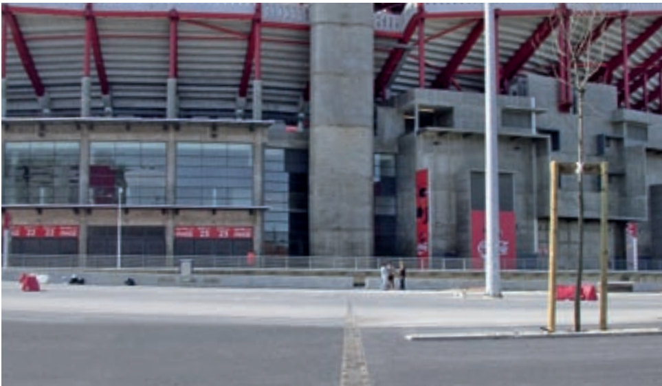
FASERFIX SUPER KS 100 Channels in front of the Estádio Da Luz in Lisbon
